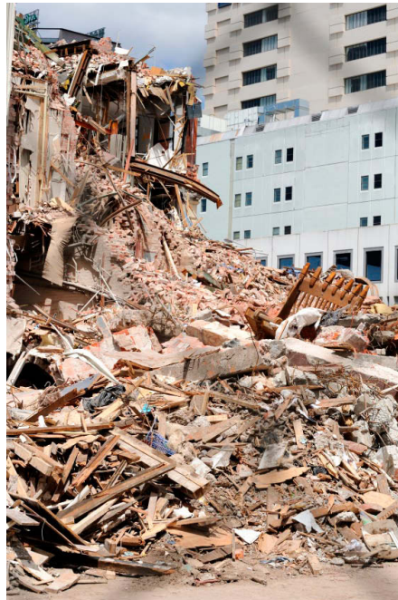
Christchurch, New Zealand - 13 January, 2011: Buildings demolished in Manchester Street. istockphoto.com.
